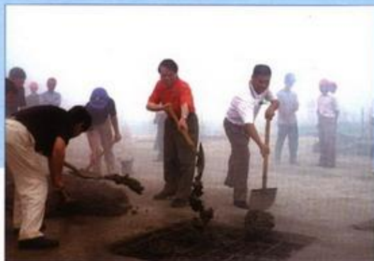
领导和嘉宾为大楼封顶
